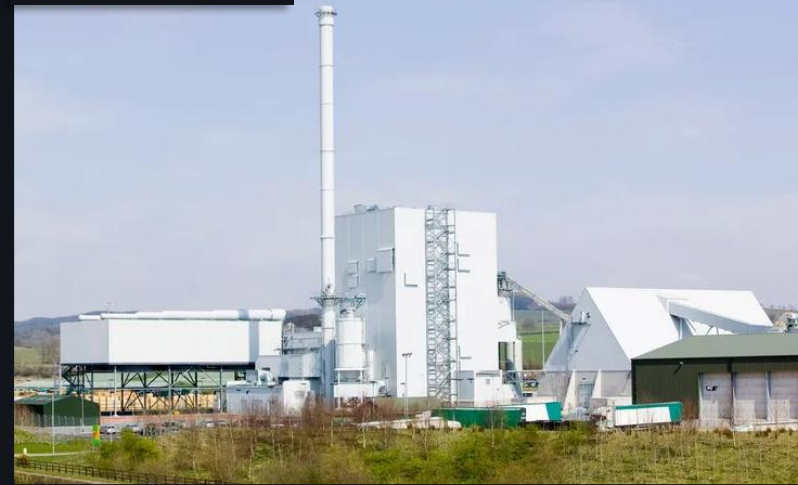
E.ON's biomass power plant near Lockerbie, Scotland, where the e-methanol project will be built. (Photo: Construction Photography/Avalon/Getty)
